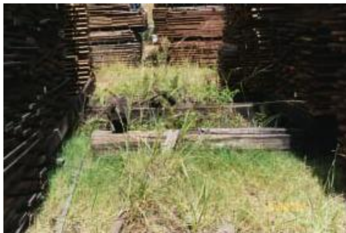
Figure 8.44. Long grass reduces airflow under racks and promotes decay and uneven drying
