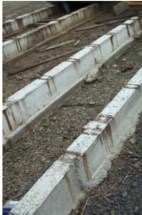
Figure 8.22. Fixed concrete kerb
