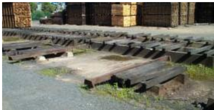
Figure 8.23. Accommodating more than two rows of stacks on concrete kerbs
