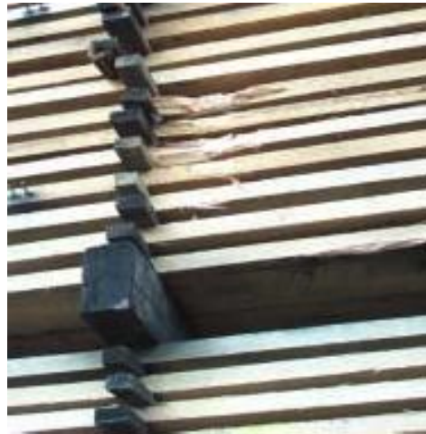
Figure 8.40 Forklift damage to a rack
