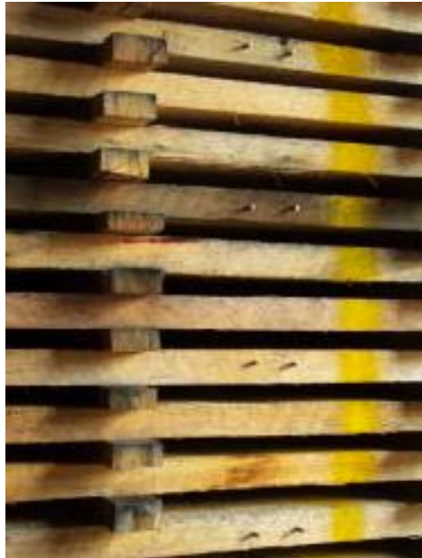
Figure 16.04. Row of testing points for a resistance moisture meter
