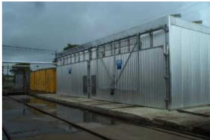
Figure 11.06. Modern final drying kiln built of aluminium clad insulated panels
