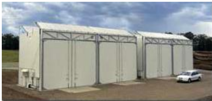
Figure 9.15. External solar collector type predryer Photo courtesy of Solar Dryers Australia
