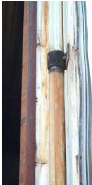
Figure 11.11. Kilns seals need to be inspected regularly and repaired as required
