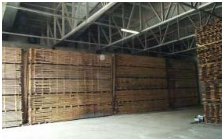
Figure 9.16. Inside a large zone predryer
