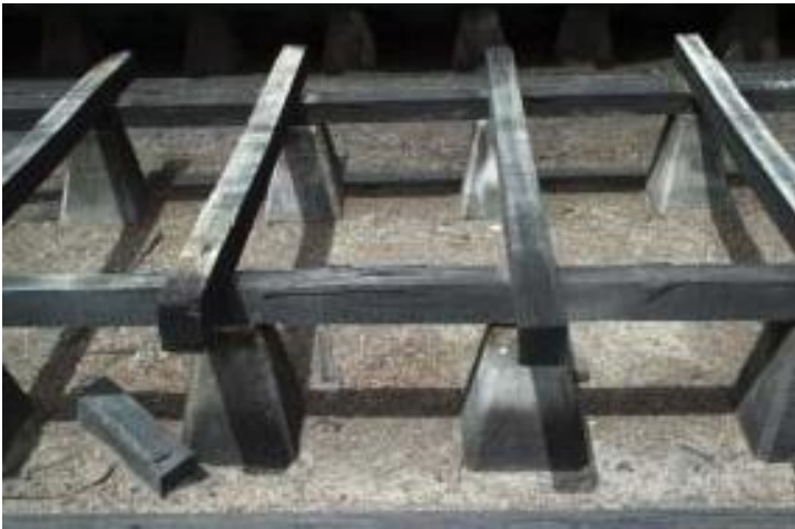
Figure 8.20. Precast concrete stack piers, with timber stringers and bearers
