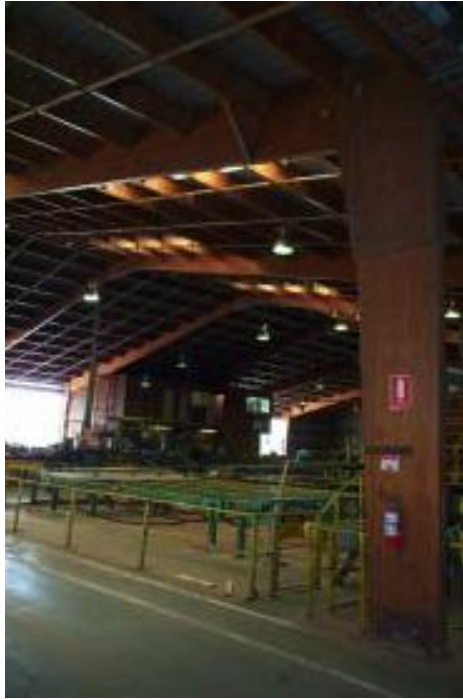
Figure 12.07. A large dry mill building
