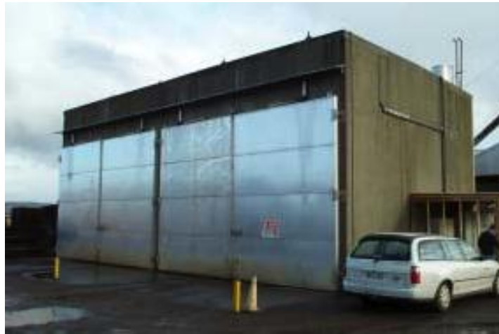
Figure 11.07. Modern precast concrete final drying kiln
