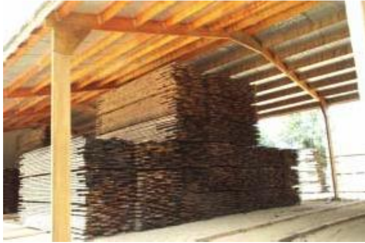
Figure 11.09. An open dry storage shed for kiln dried material awaiting transport to the dry mill
