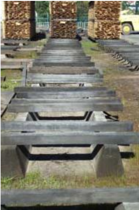
Figure 8.21. Fixed concrete kerb with bearers
