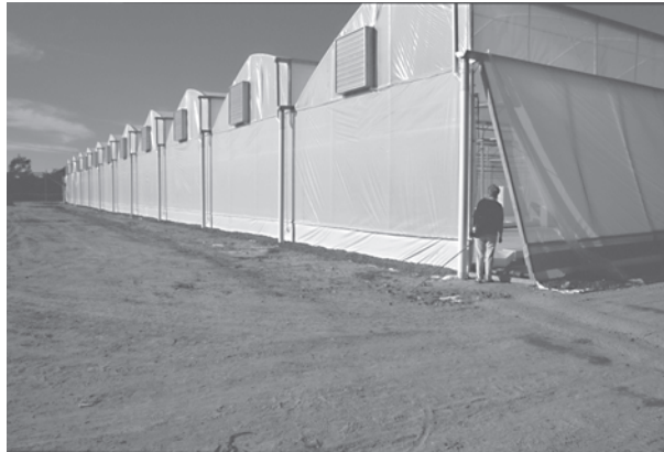
Sidewall screening is an effective way of excluding pests from the greenhouse
