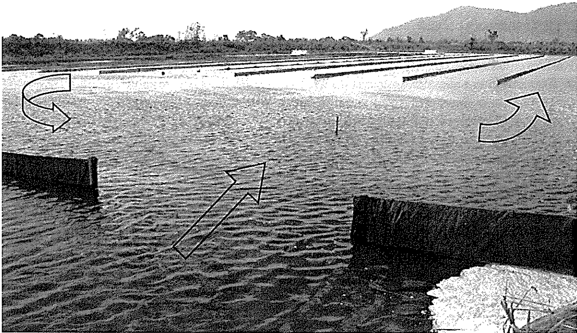
Figure 2.4 Overflow gate and bioremediation zone of treatment pond, showing direction of water flow.
