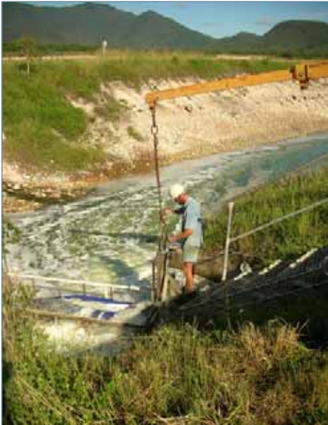
Figure 7.2 Drain harvesting with a harvest cage
