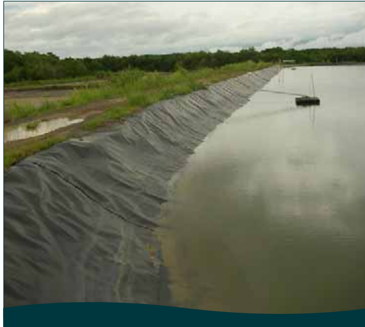
Figure 2.2 HDPE black plastic liner installed on a pond wall to minimise erosion from wind action and rain
