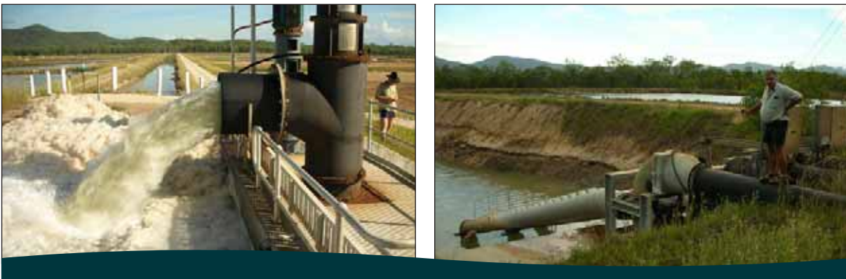
Figure 2.6 Typical prawn farm intake pump systems
