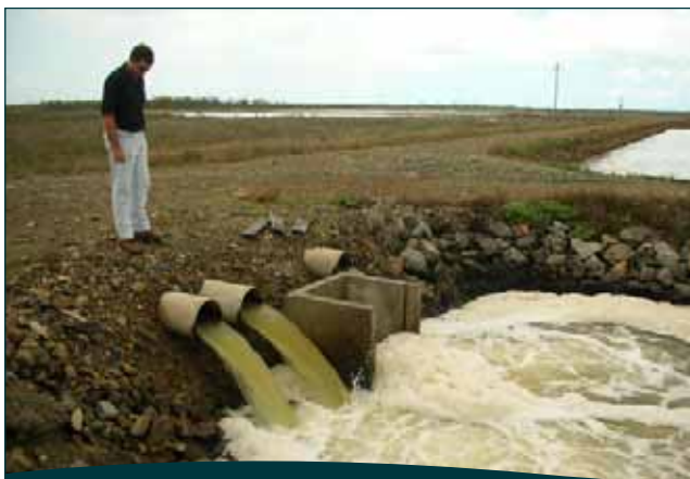
Figure 2.13 Using recycled water to fill new ponds (note the green algae colour)
