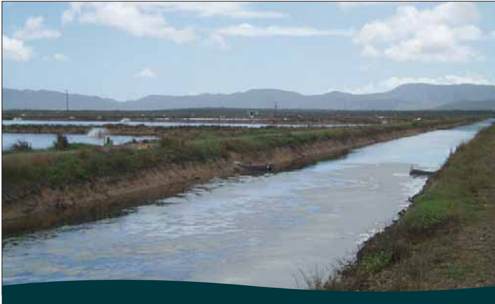
Figure 2.7 An aqueduct channel delivering water to the growout ponds
