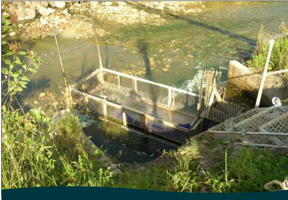
Figure 2.9 Harvest cage installed at the pond outlet
