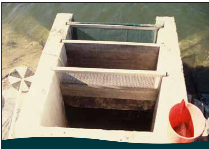
Figure 2.4 A 'monk' water control and outlet structure
