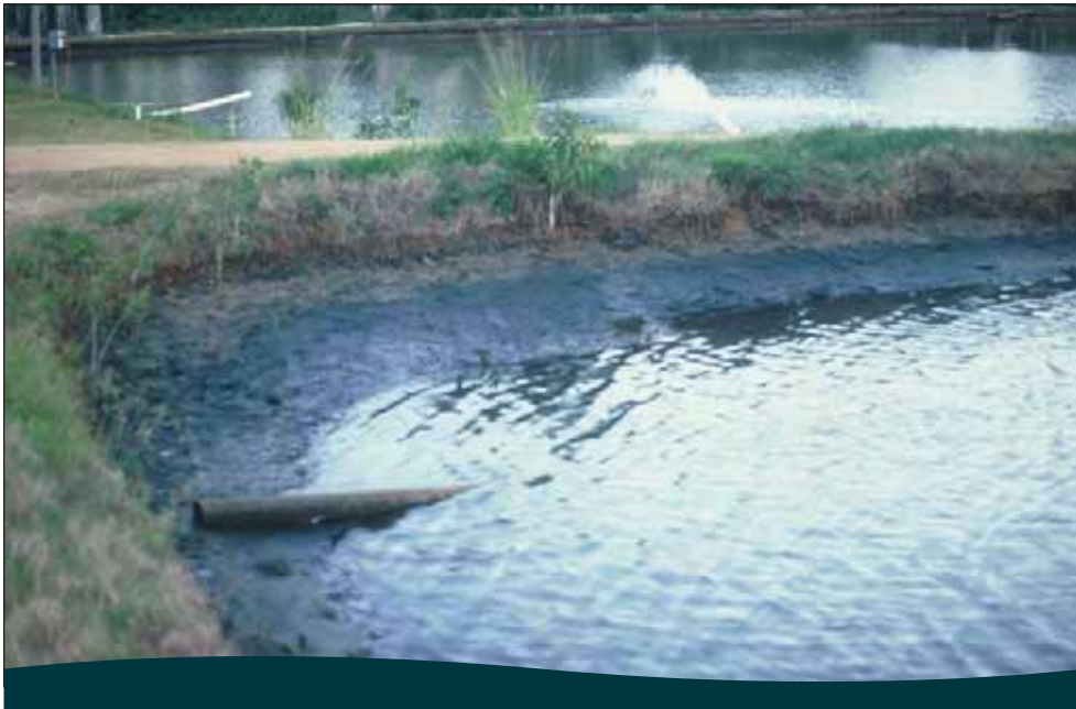
Figure 5.8 Mats of dead algae deposited in a windward corner
